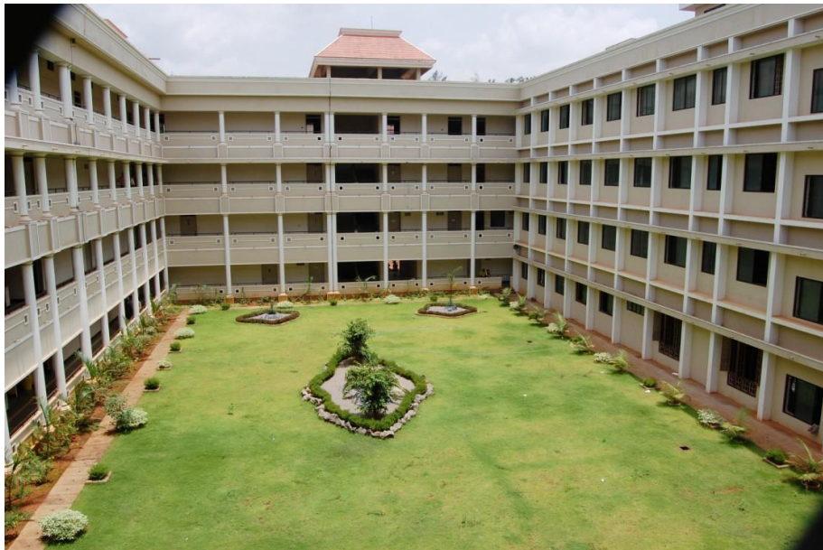
Inner View of Main Block
